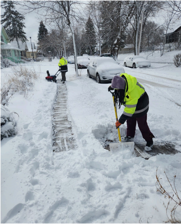
Figure 3: Minneapolis Snow Ambassadors clearing priority sidewalks during the 2024-2025 pilot program. Manual labor with shovels and walk-behind blowers remains the standard approach.
